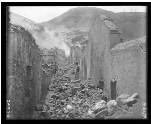
Left: Rubble covers a side street in northern Saint-Pierre in 1902.
